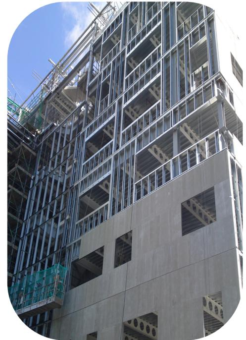
*Steel Framing used to form a Rapid Dry Envelope (RDE)*
