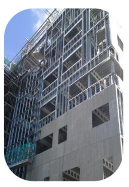
Steel Framing used to form a Rapid Dry Envelope (RDE)
