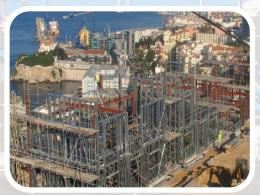
system, which is fixed as a rapid dry infill between the main structural frame members. The system acts as a carrier for external cladding, internal wall make-up and insulation. ASF is designed to suit the loading, deflection dimension requirements of each project. The cold rolled galvanised framing consists of
